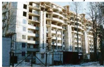
Fig. 3. Moscow, 2002. Building at 4 Khimkinskiy Bul'var – vertical extension in progress [15]
